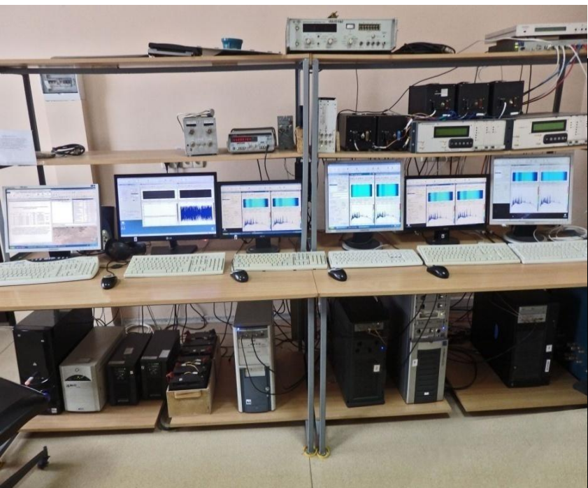
Fig. 23. The equipment room UTR-2 - GURT with back-end facilities of new generation.
